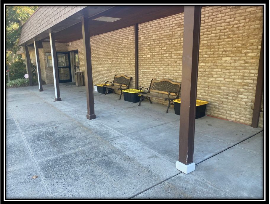
Columns – The white areas are the repaired areas that will later get painted.
